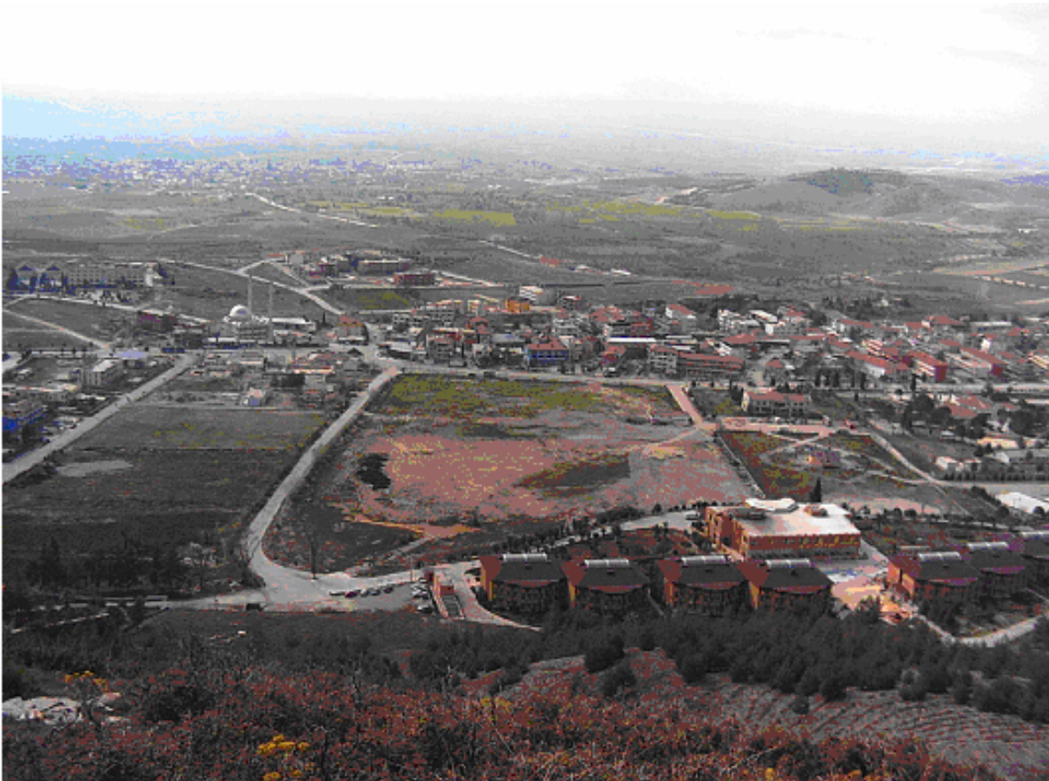
The Project Site of Spa Treatment Center
